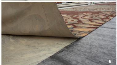
Once prescribed open time is allowed, install the carpet into the adhesive, peeling back a section periodically to make sure the adhesive is penetrating into carpet-backing recesses (figures D and E).
