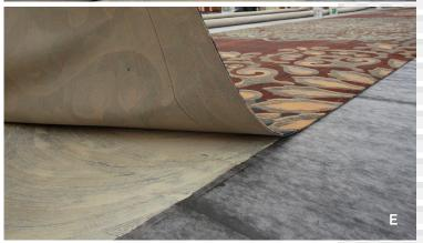
Once prescribed open-time is allowed, install the carpet into the adhesive, peeling back a section periodically to make sure the adhesive is penetrating into carpet backing recesses (figure D and E).
